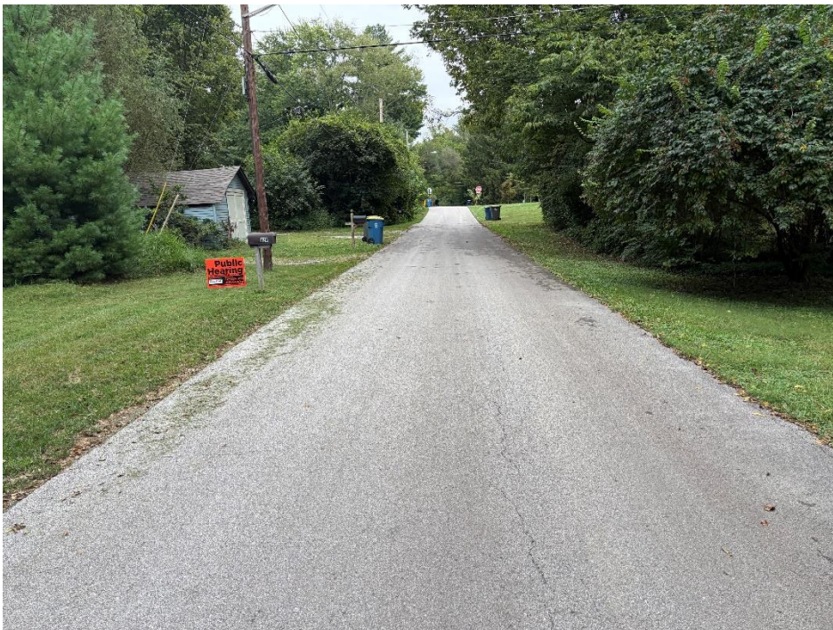
Subject Site: Facing West on W 54 th Street
