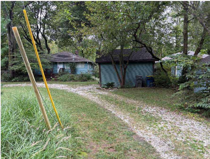
Subject Site: Facing north. Existing utility shed and driveway. Limited access to rear yard
