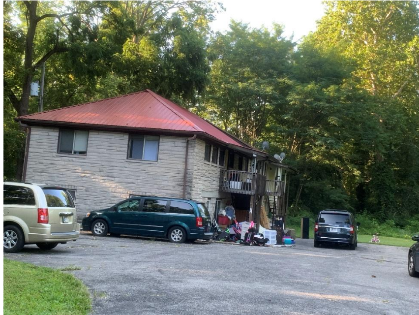
Photo 5: Multi-Family Building (Southeast Building) Viewed from North
