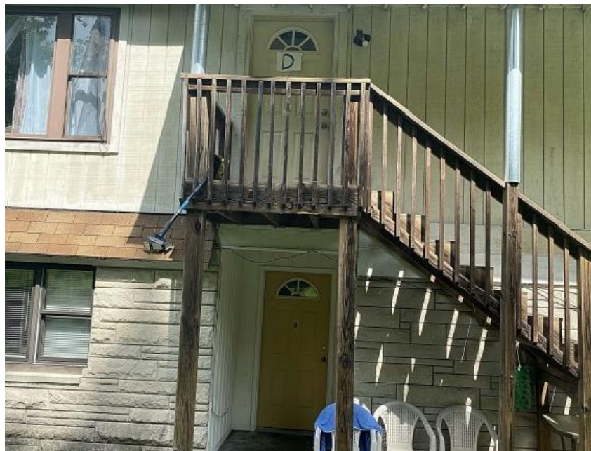
Photo 8: Entrances to Units B and D of Multi-Family Building Viewed from East
