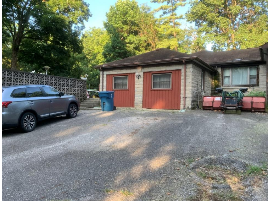
Photo 3: Single-Family Residence (Northwest Building) Viewed from East
