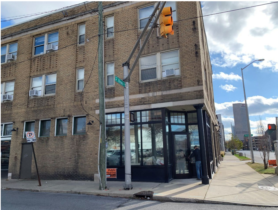
Photos of the subject building (top); and tenant space entrance of the proposed tattoo parlor
