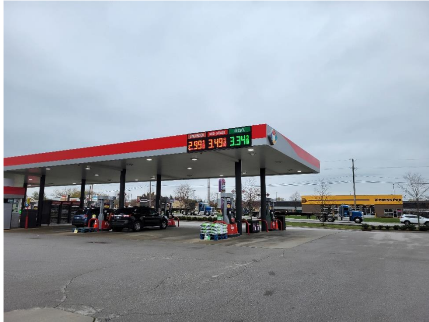
Photo 3: Existing Digital Price Display on Northern Elevation (to remain)
