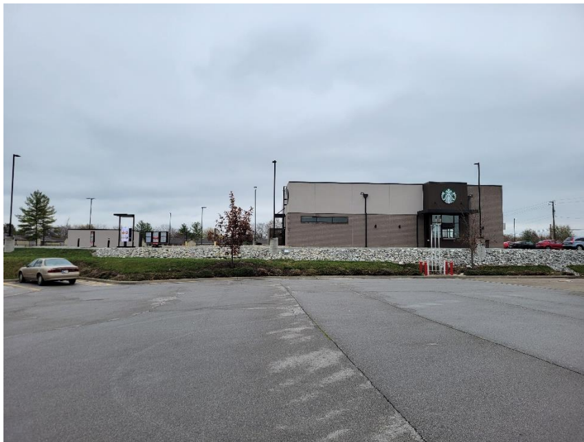
Photo 8: Adjacent Property to East
