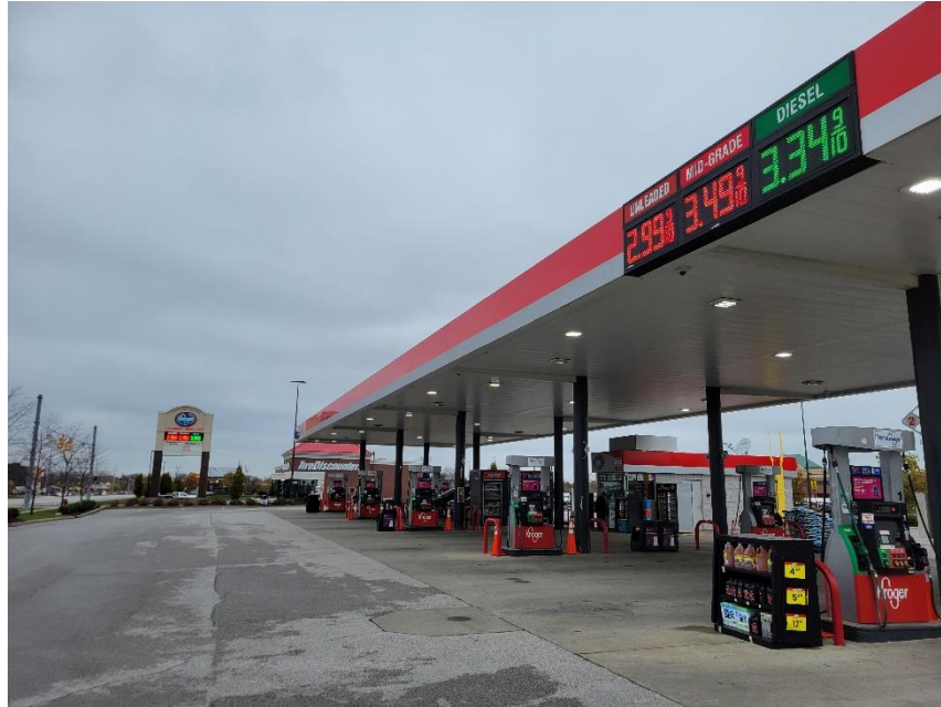
Photo 1: Existing Pump Island Canopy & Pylon Sign
