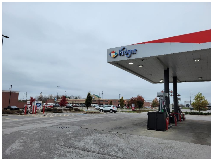
Photo 6: Existing Tenant Signage on Northern Elevation
