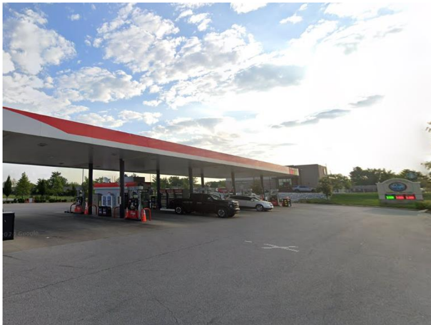
Photo 2: Existing Pump Island Canopy & Monument Sign (taken September 2024)
