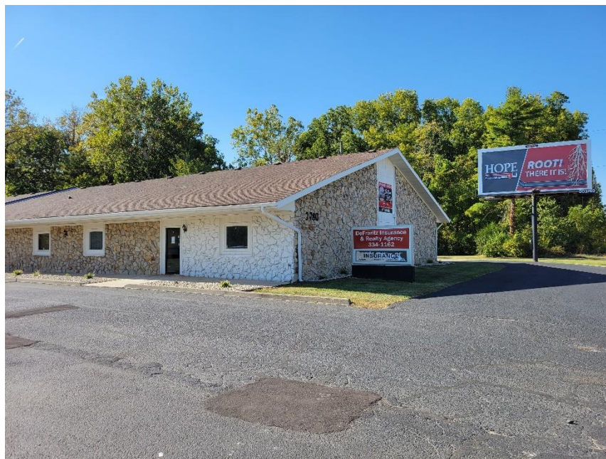
Photo 2: Subject Site viewed from Southeast
