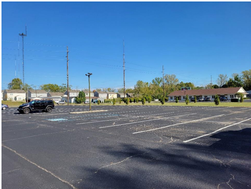
Photo 8: Parking Area for Full Multitenant Center
