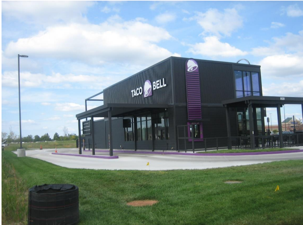
Existing outlot development with two of three wall signs, looking northeast
