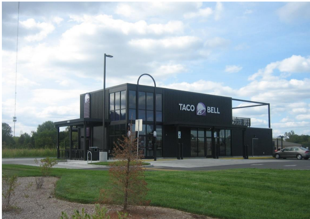
Existing outlot development with two of three wall signs looking northwest
