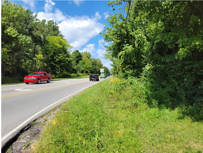
Photo 1: Sidewalk Area along Lee Road (waiver requested)
