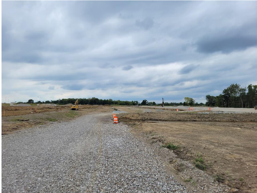
Photo 1: Subject Site Viewed from East
