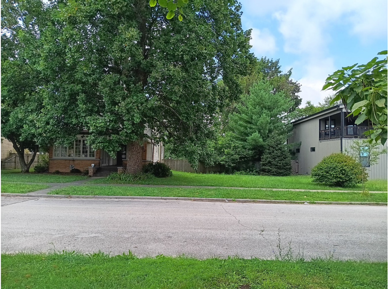
Exhibit 4: 2522 Carrolton Avenue (Left), with empty area of parcel where the two parcel divisions will occur.
