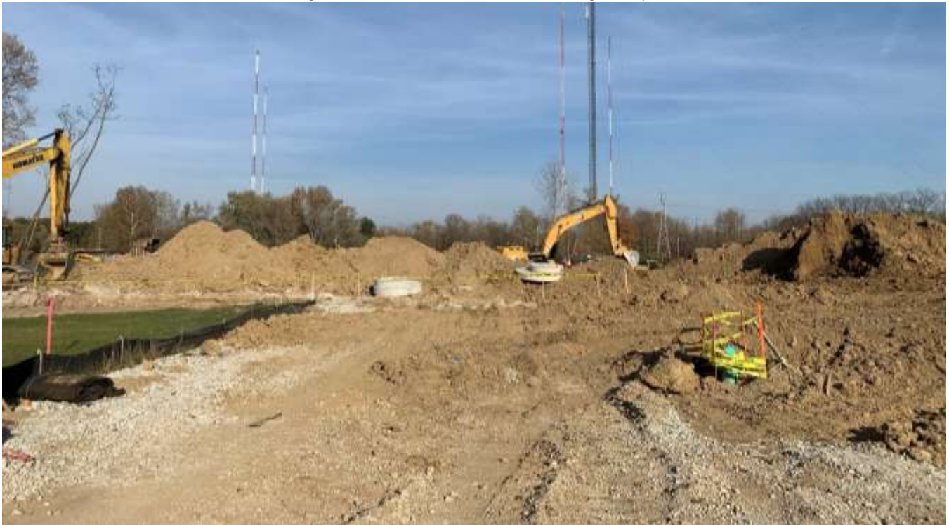
Photo looking northeast along Emerald Street from Amethyst Avenue.
