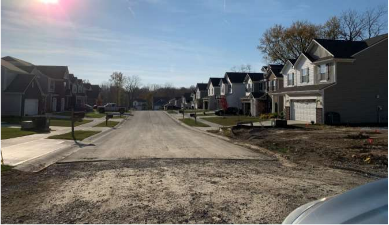
Photo looking southwest along Emerald Street from Amethyst Avenue.
