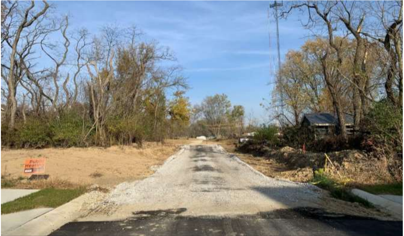
Photo looking northeast along Moonstone Street.
