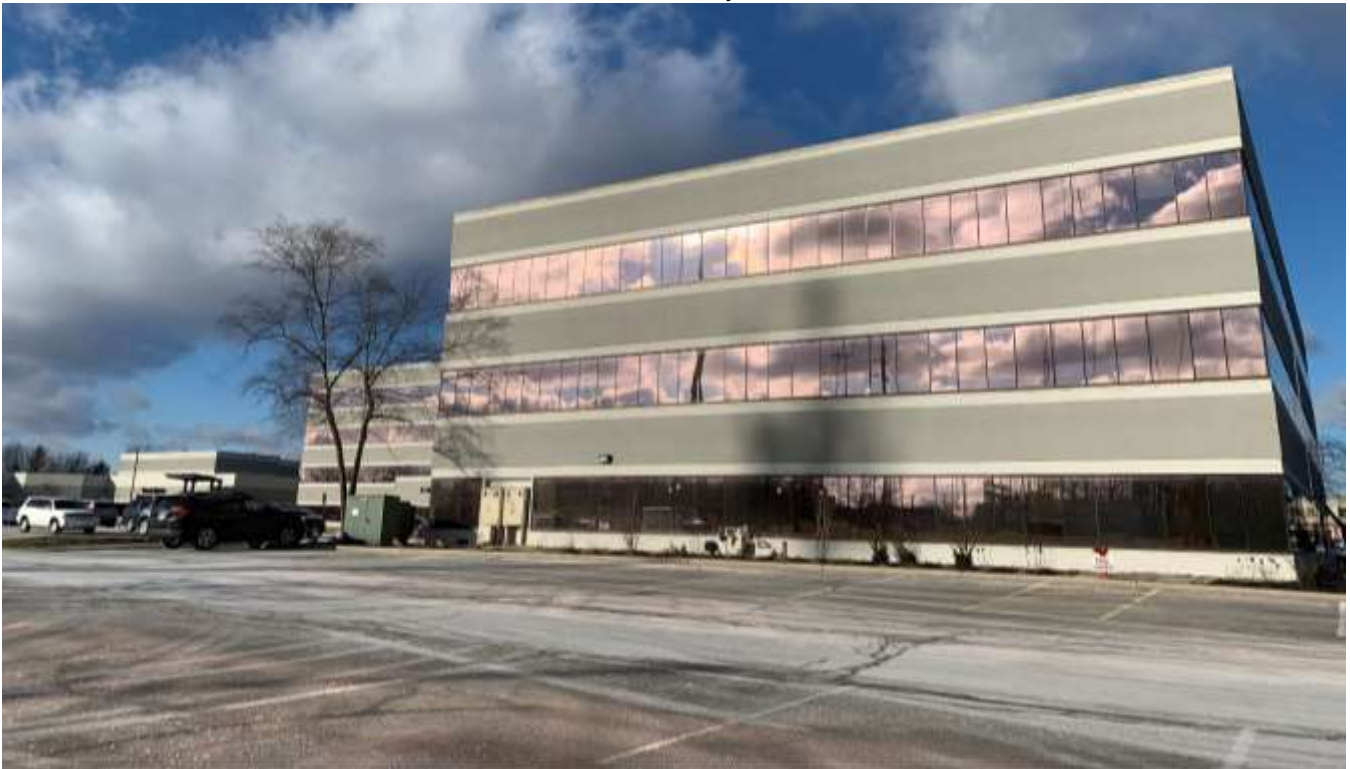
Photo of the southern building elevation where the proposed sign will be located.
