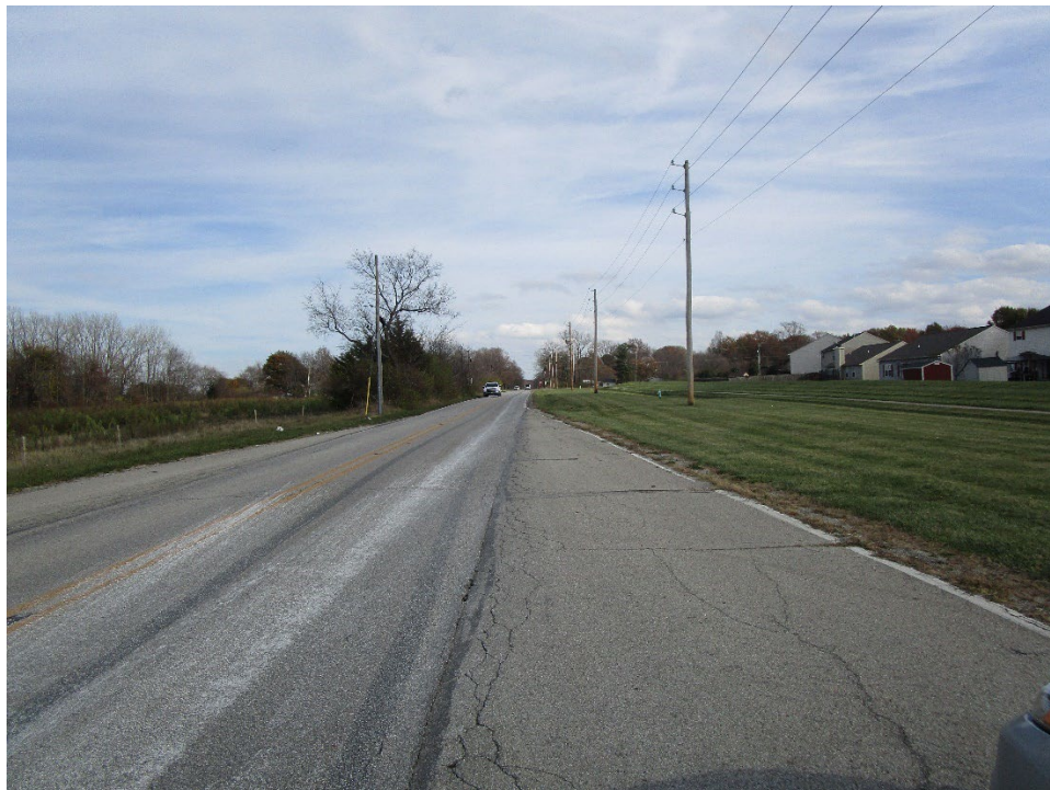
View looking east along East 38 th Street
