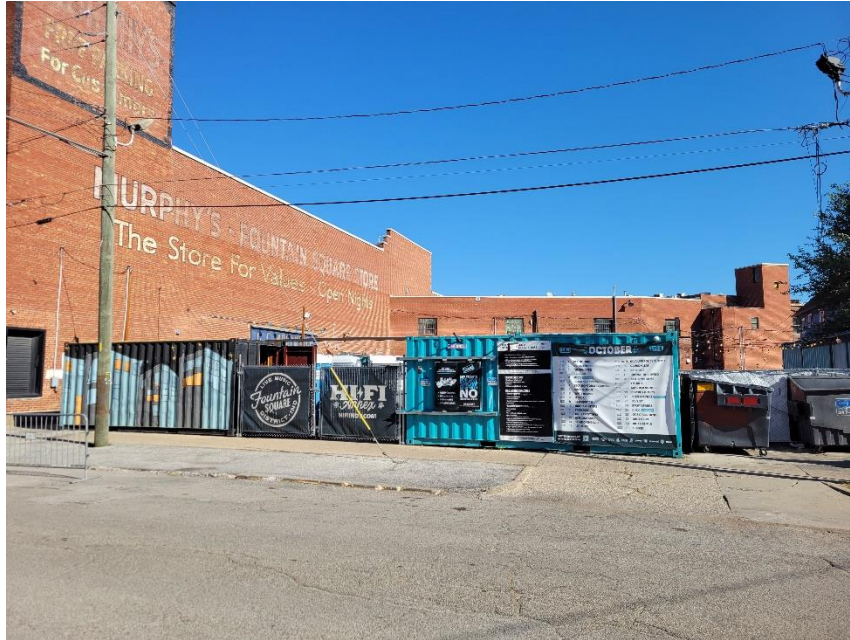
Photo 1: Subject Site Viewed from West
