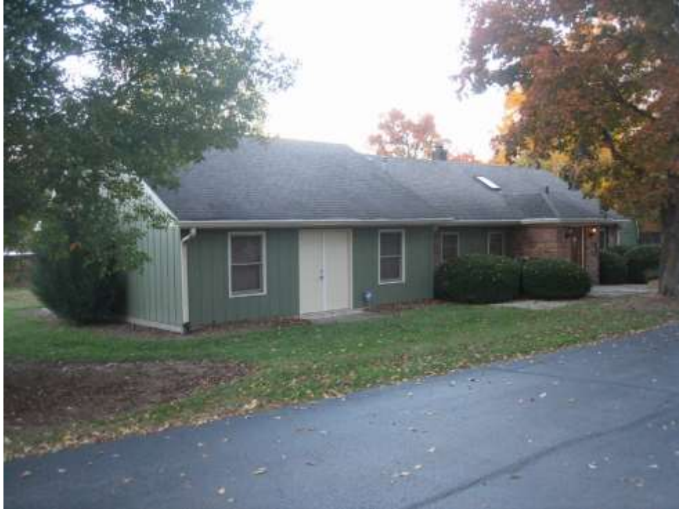
Subject site, looking northeast.
