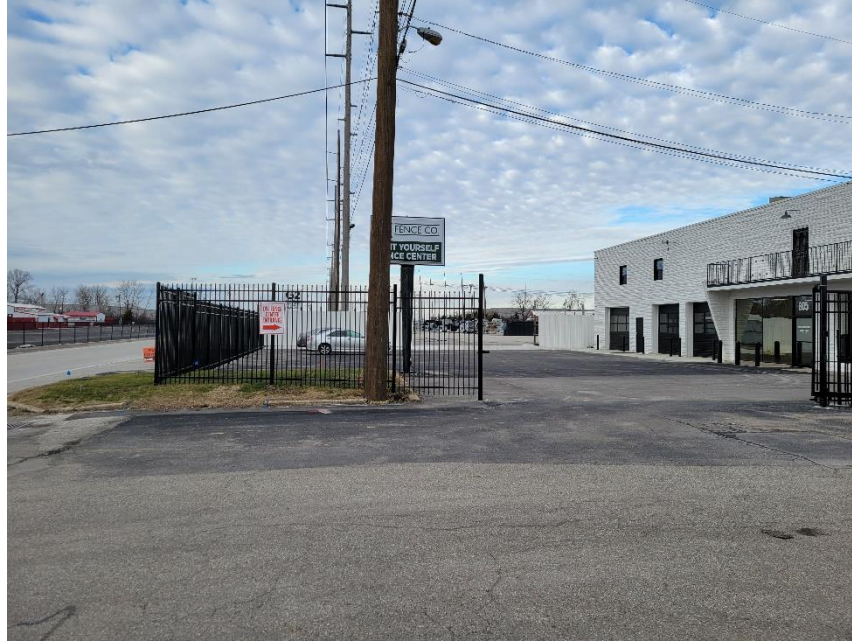
Photo 3: Fence from South
