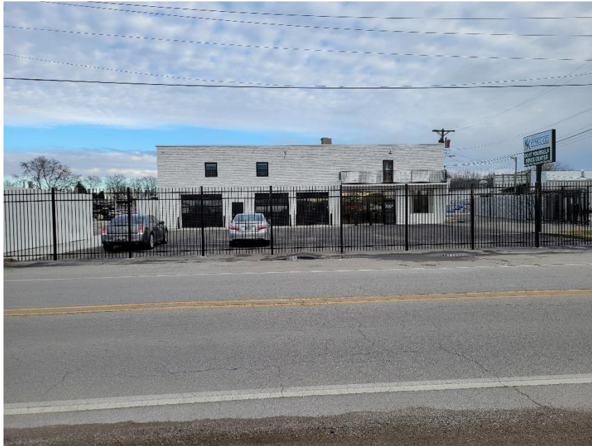
Photo 1: View of the Subject Site (from West)
