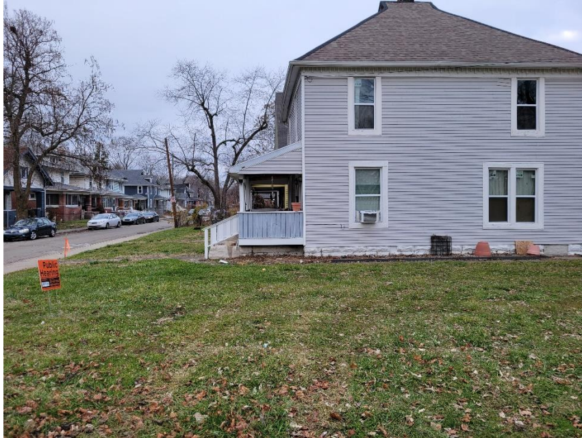
Photo 3: Neighboring Property to the North
