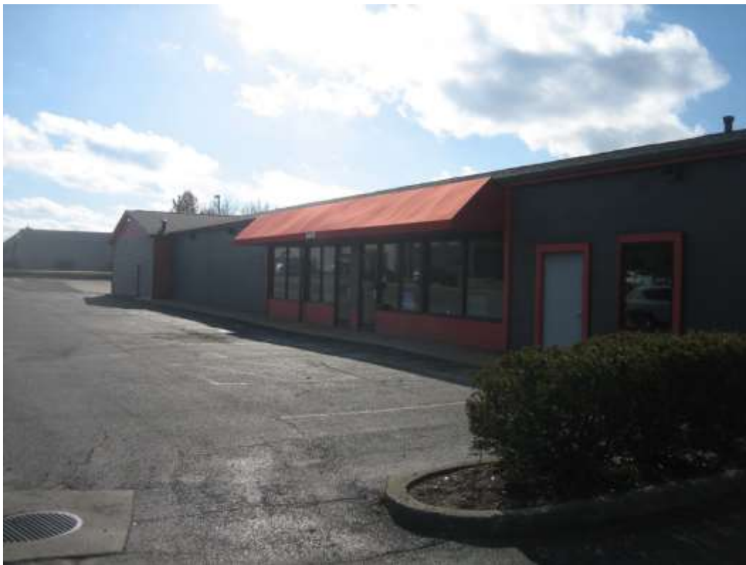
View of subject site, east side of existing building to be demolished, looking southwest
