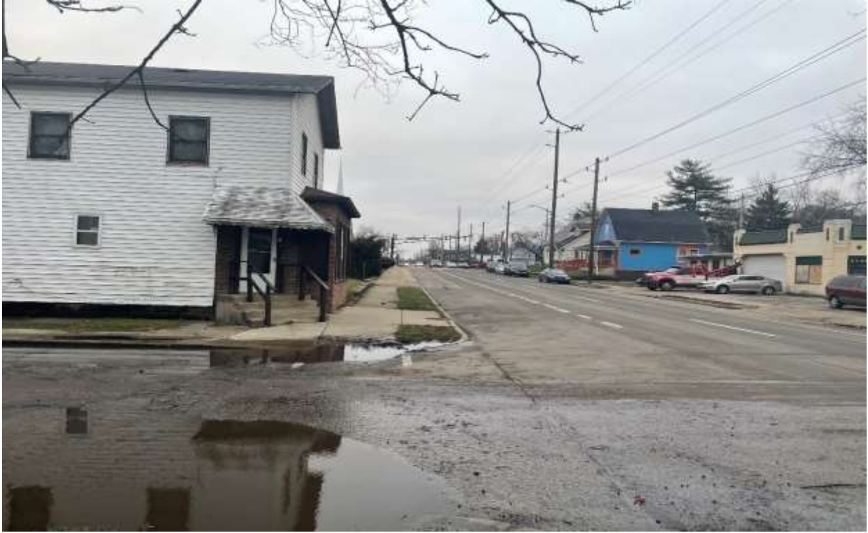
Photo One: Looking East Along Michigan Street
