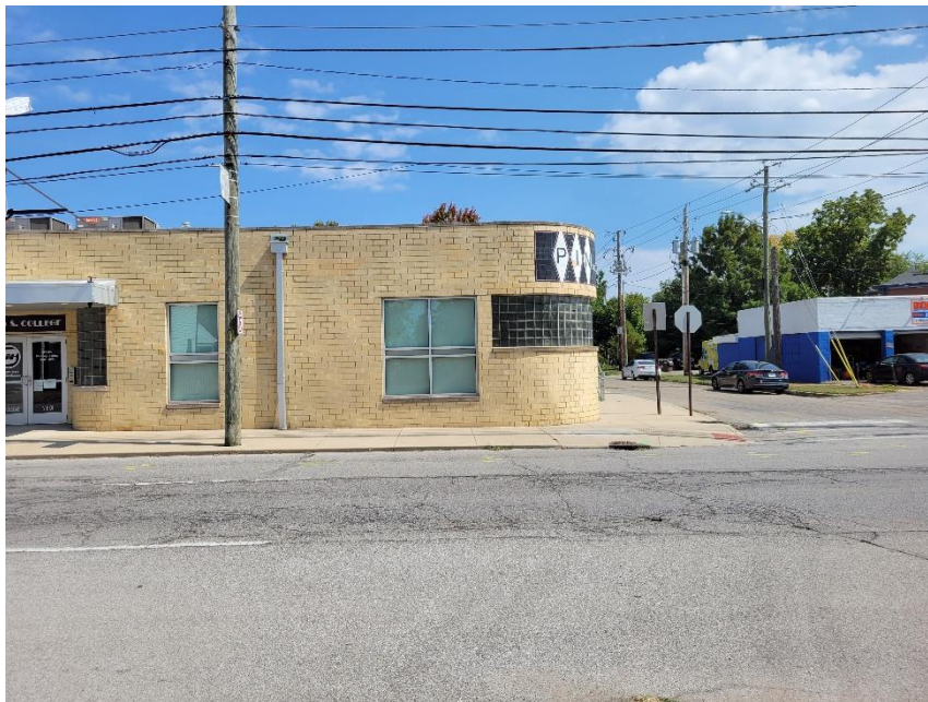
Photo 6: Adjacent Property to East
