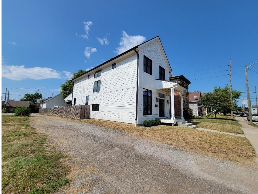
Photo 3: Alley to North and Adjacent Property Viewed from East
