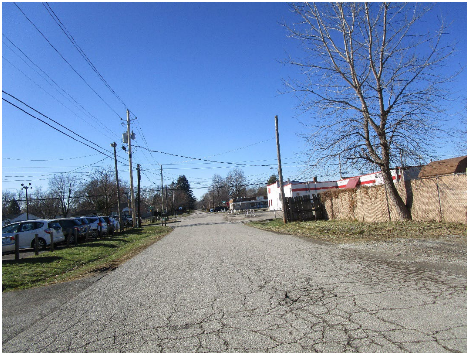
View looking west along Dudley Avenue
