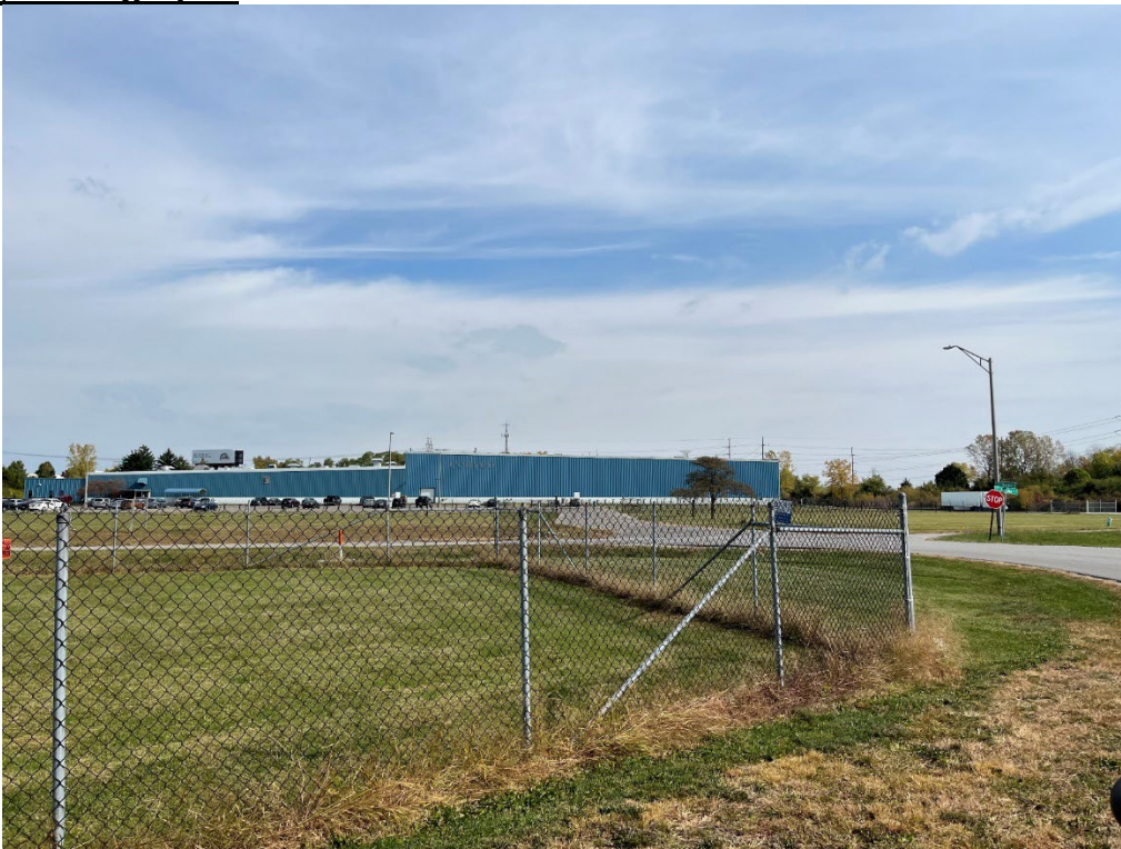
Photo of industrial property to the northeast.
