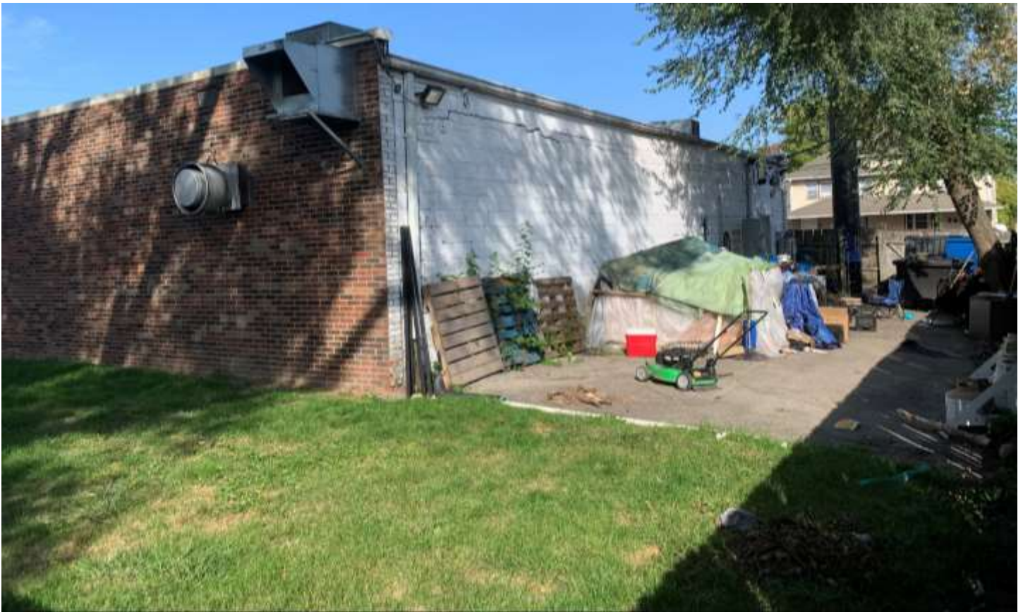
Photo of the existing east building façade looking north.
