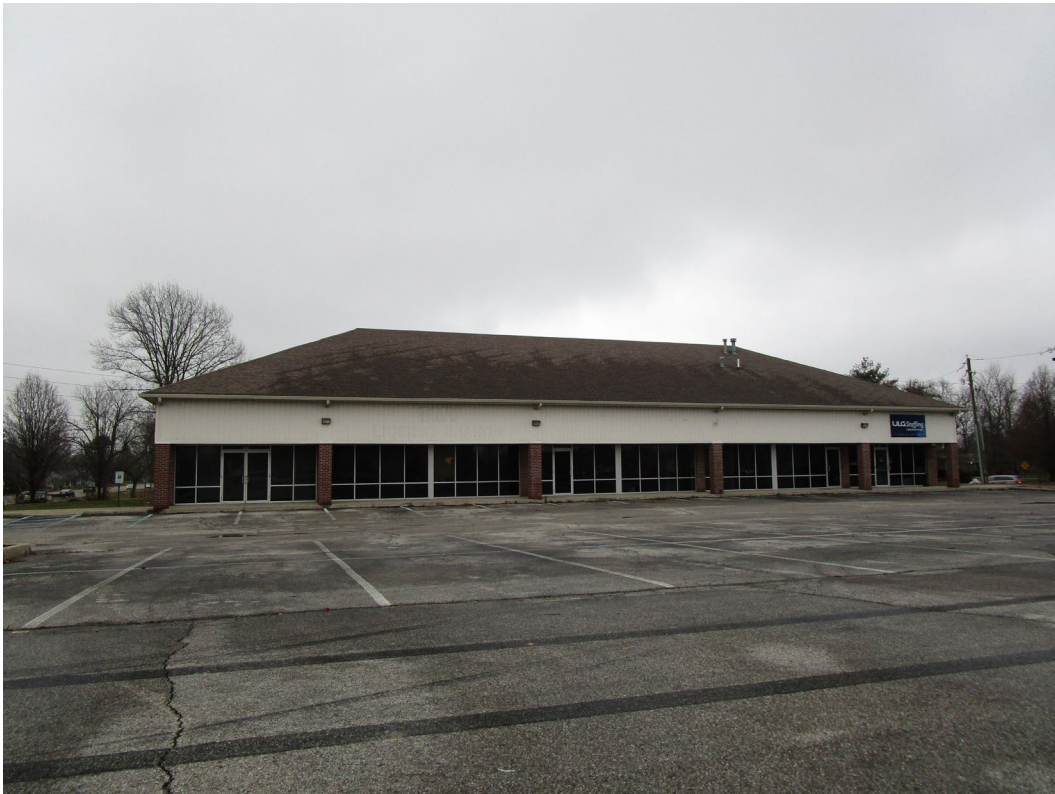
View existing building proposed for redevelopment of a convenience store
