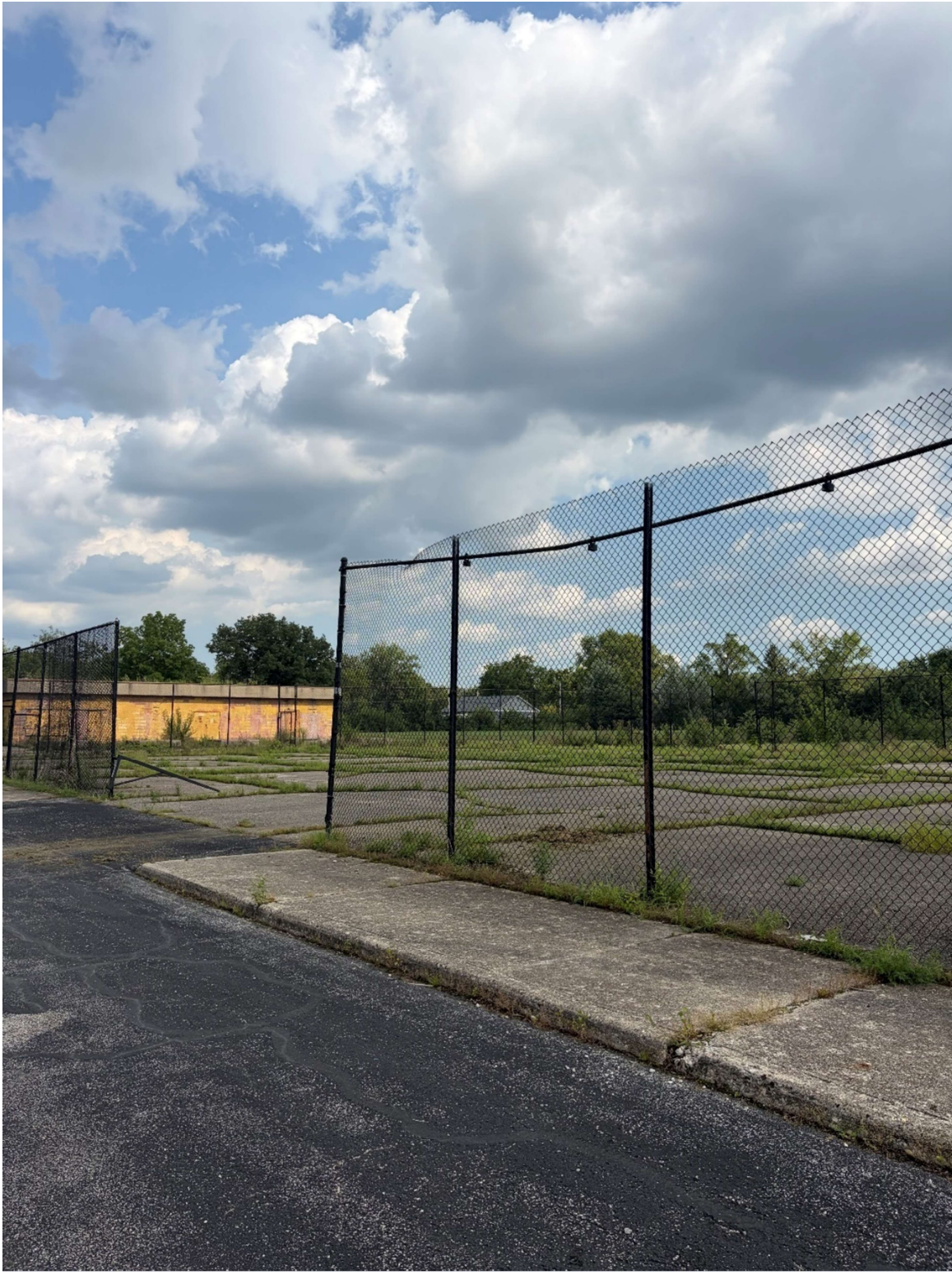
Looking East towards building adjacent to proposed site and field
