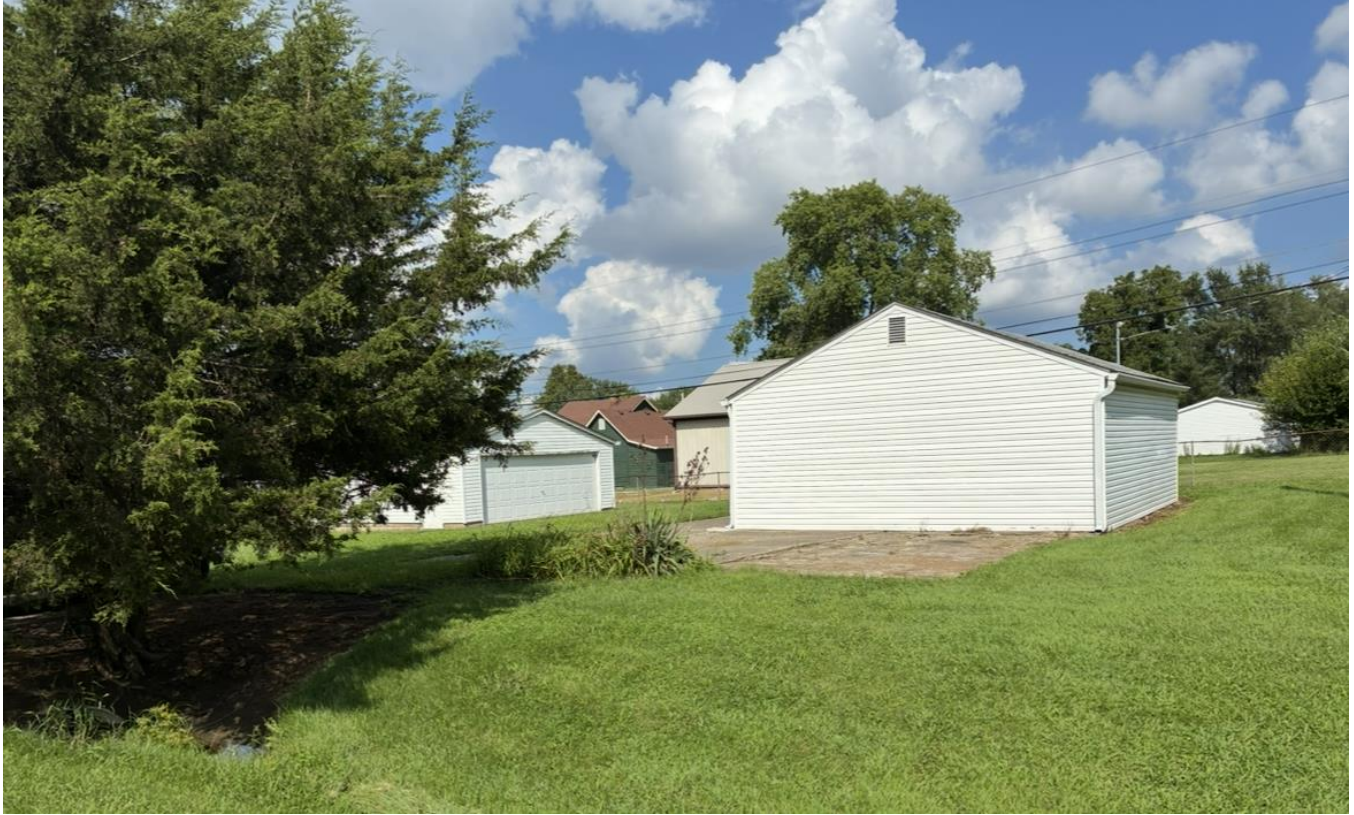
View of existing accessory garage structures from Keystone Ave
