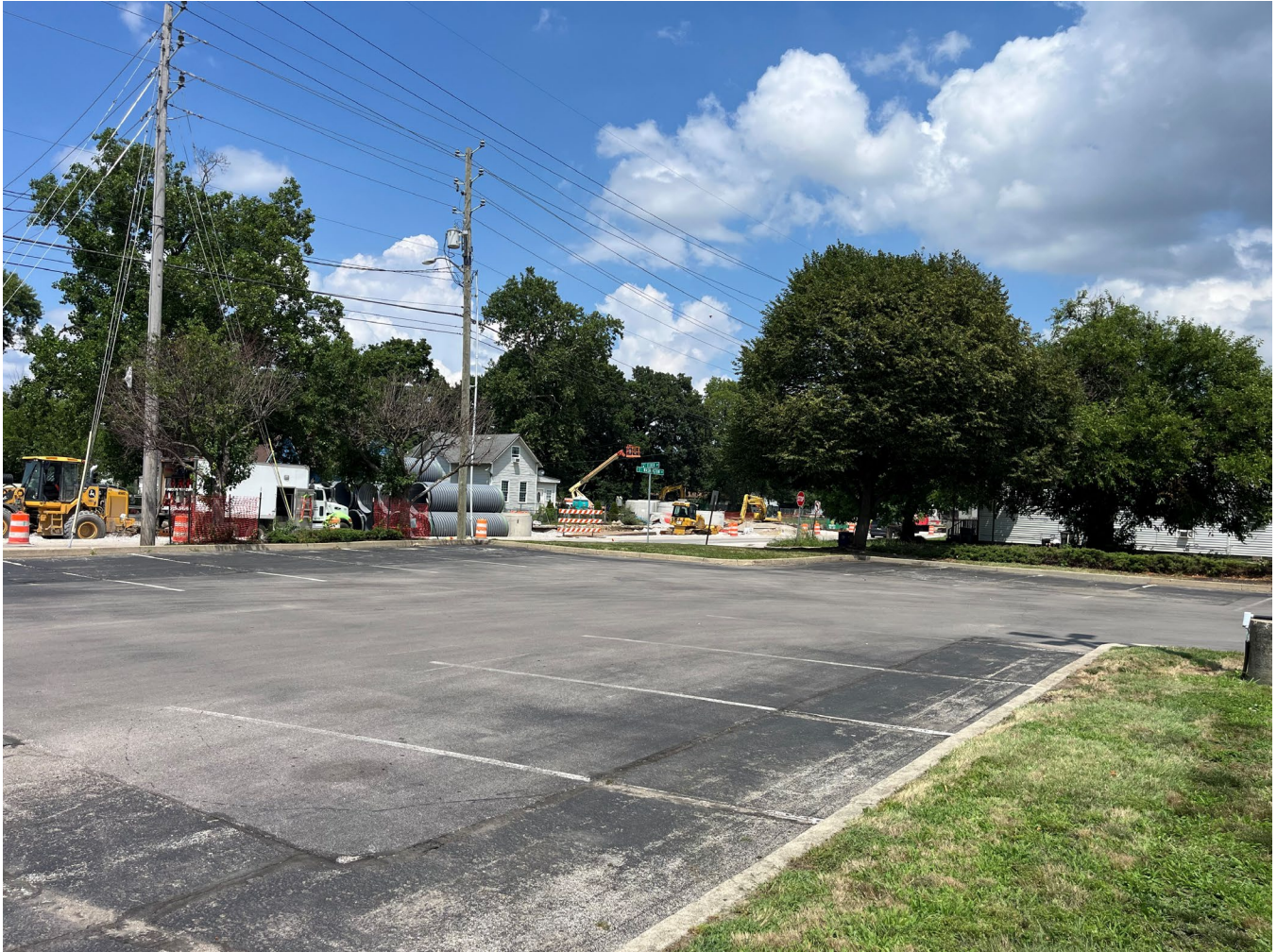
Photo 5: Reconstruction of Washington Street to support Blue Line Bus Rapid Transit can be seen in background.
