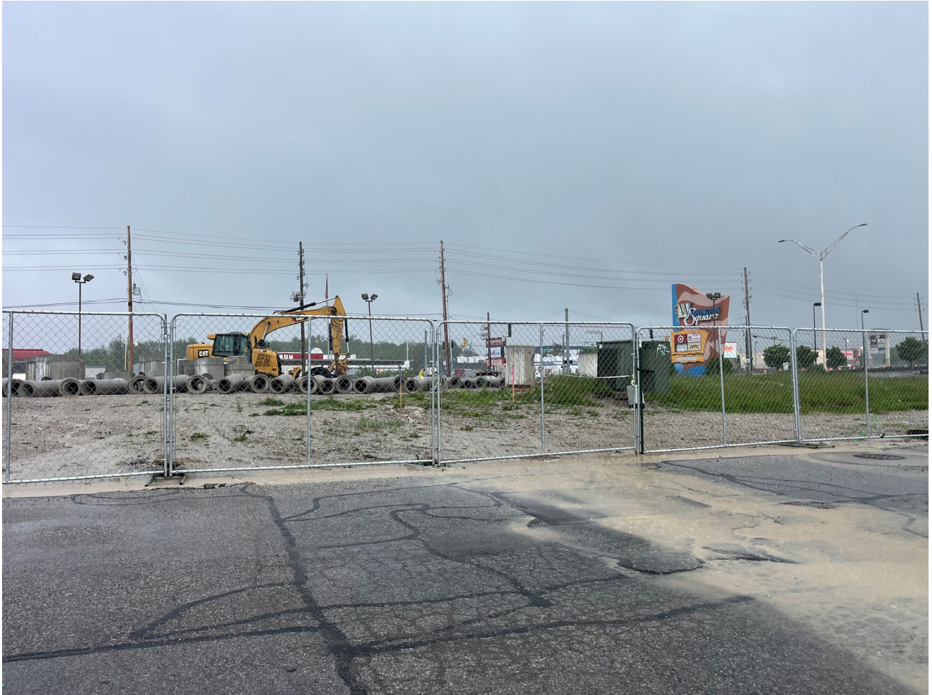
Photo 1: Subject site from mall parking lot
