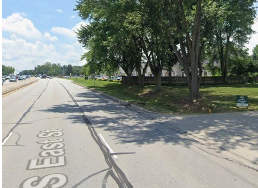
Photo 3: Potential Sidewalk Area to South of Driveway (June 2025)
