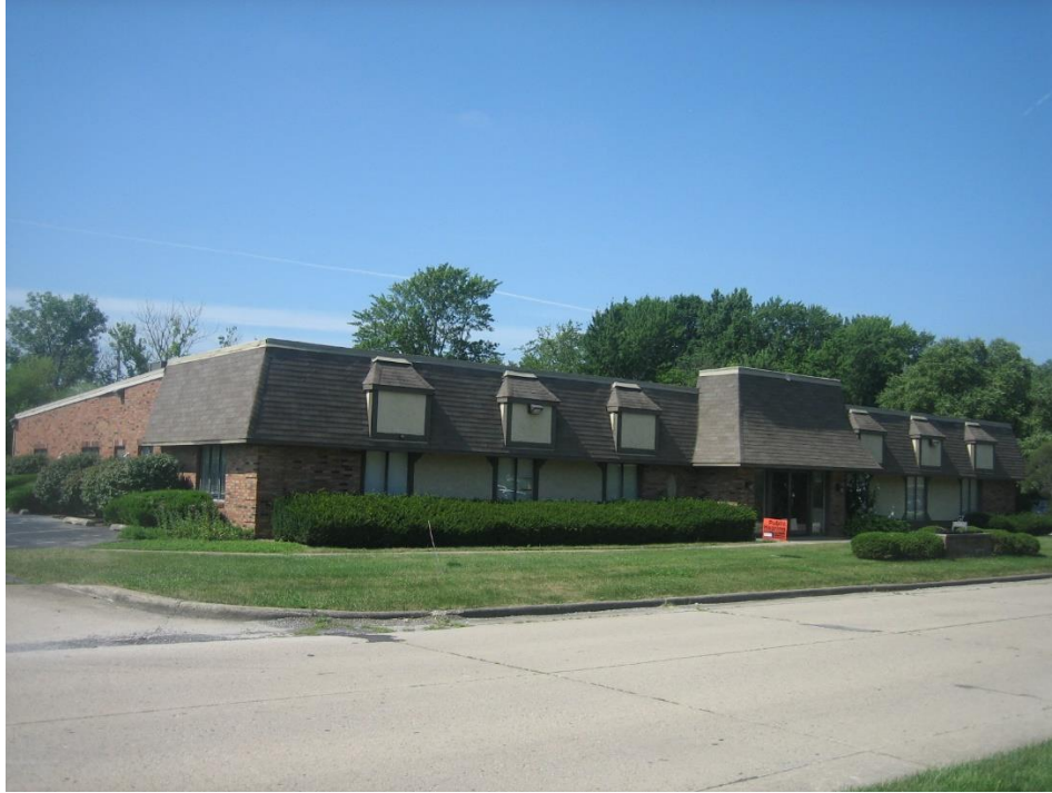
Subject site, looking south.
