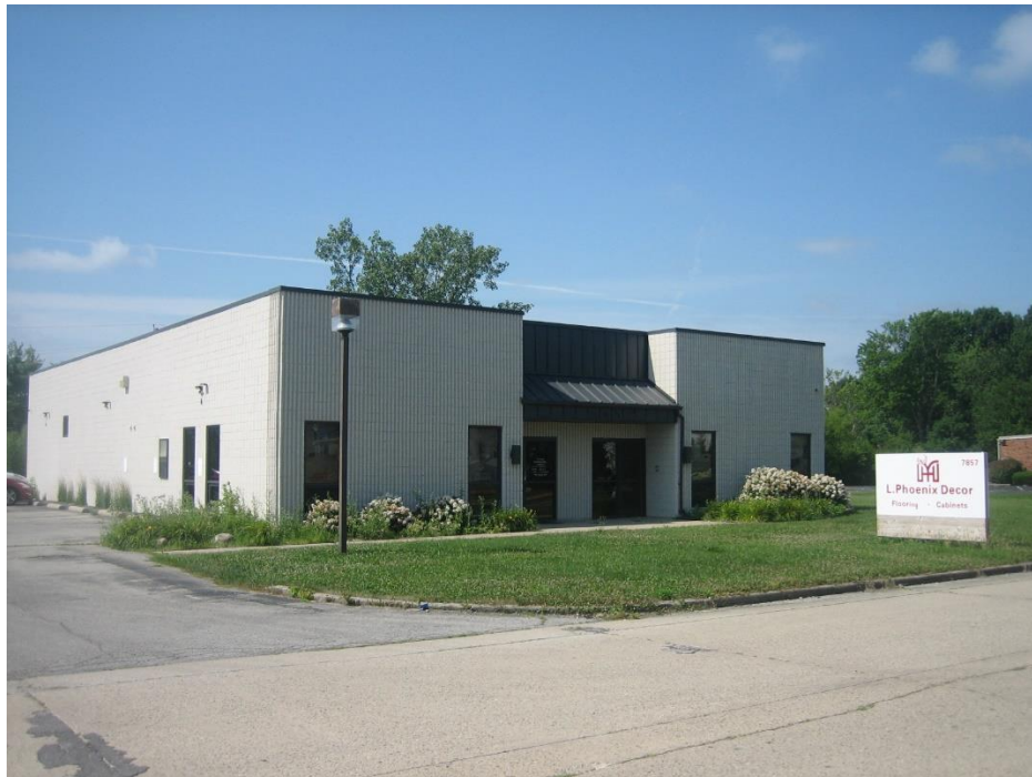
Adjacent office use to the east, looking southwest.
