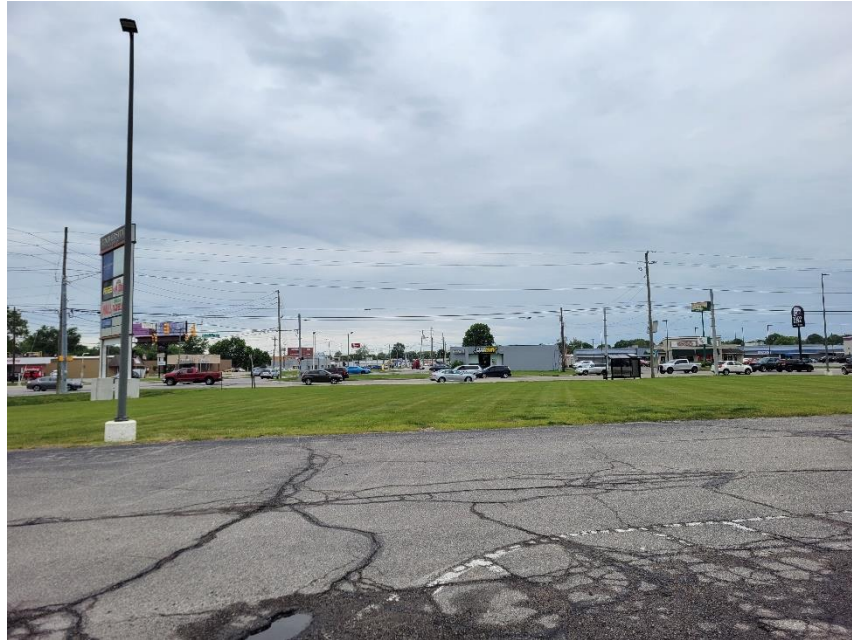
Photo 1: Subject Site Viewed from East
