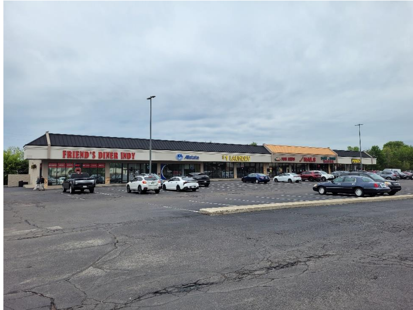
Photo 7: Adjacent Property to North
