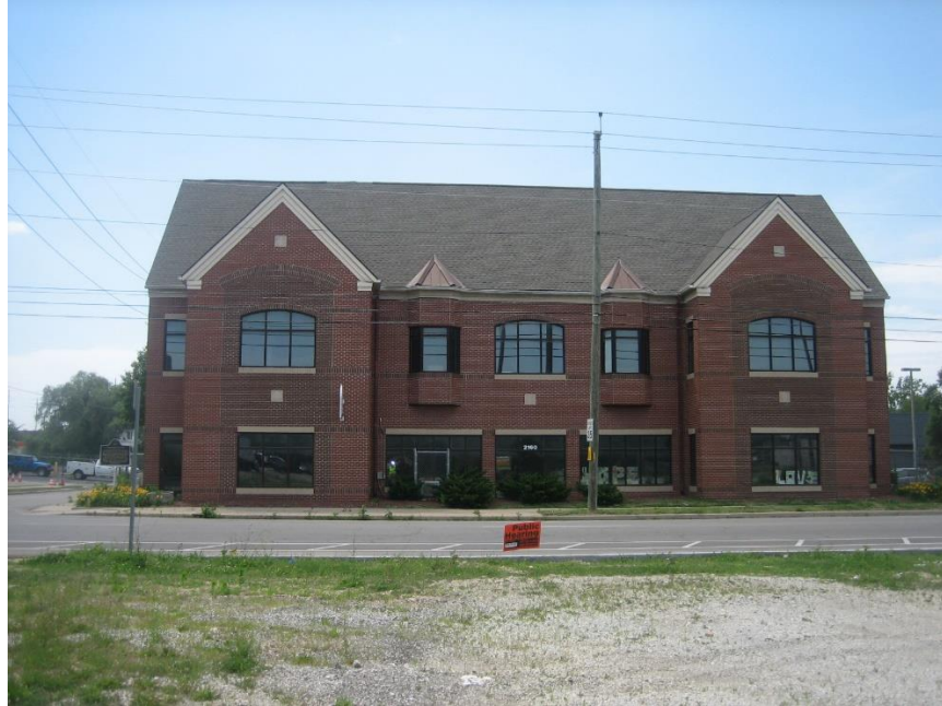
Adjacent office commercial use to the west.
