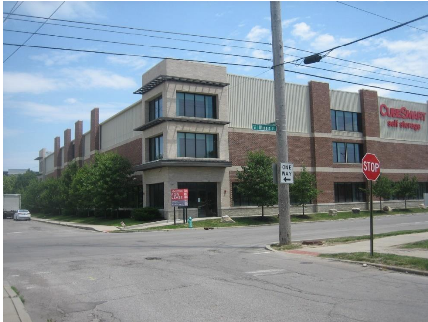
Adjacent self storage to the south, looking southeast.
