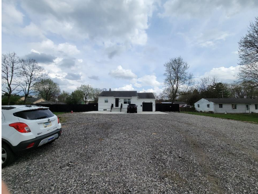
Photo 1: Subject Site Viewed from West
