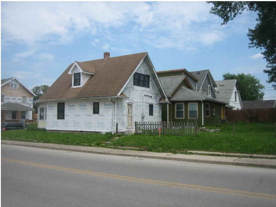
Single family dwellings to the east of subject site.
