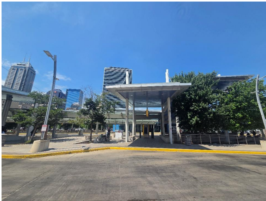
Photo 12: Adjacent Property to North
