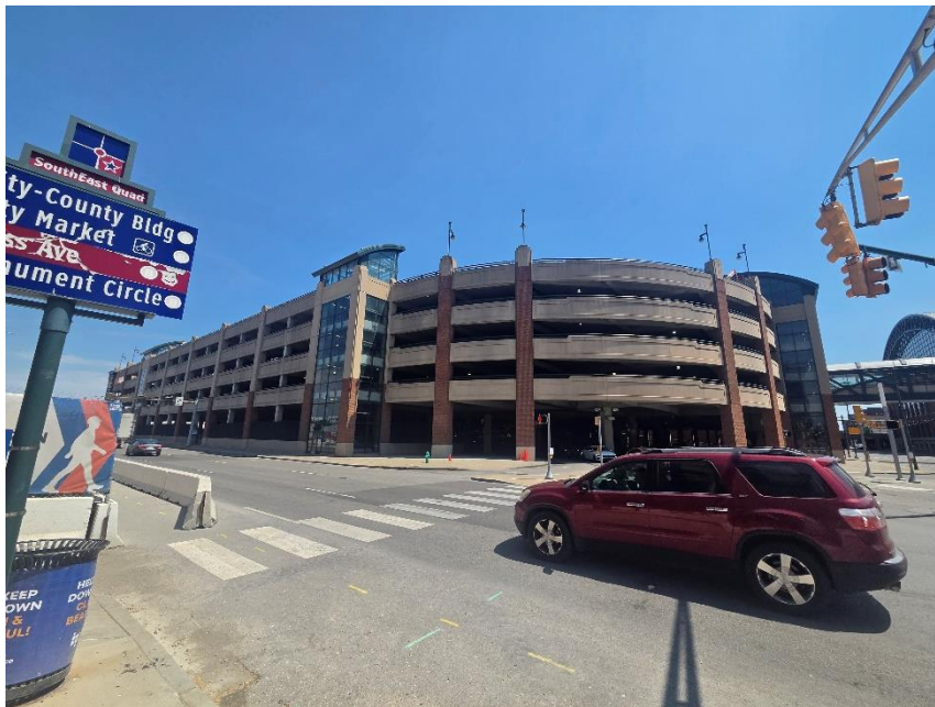
Photo 10: Adjacent Property to South (viewed from west)
