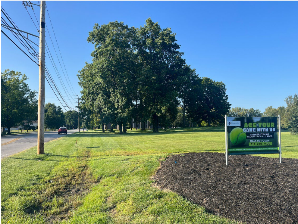
Looking south along the North-South portion of Guion Road
