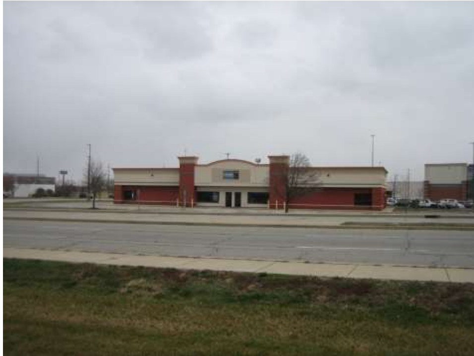
Subject site existing building to be demolished, looking north
