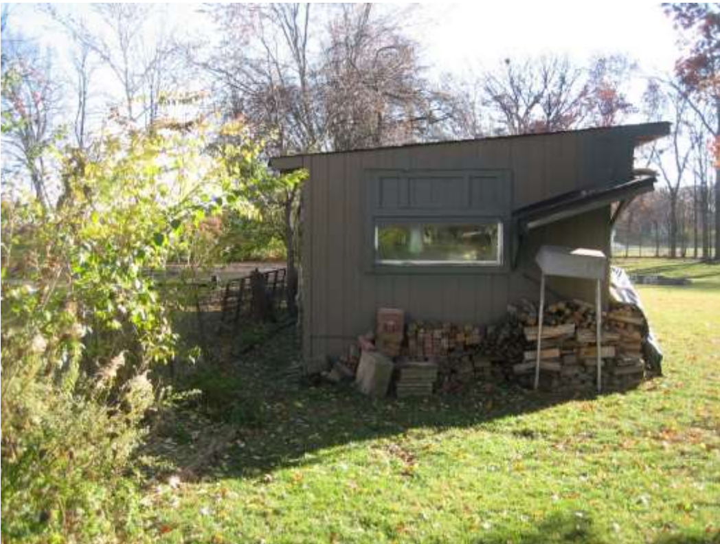
The east side property line, and shed setback, looking south.
