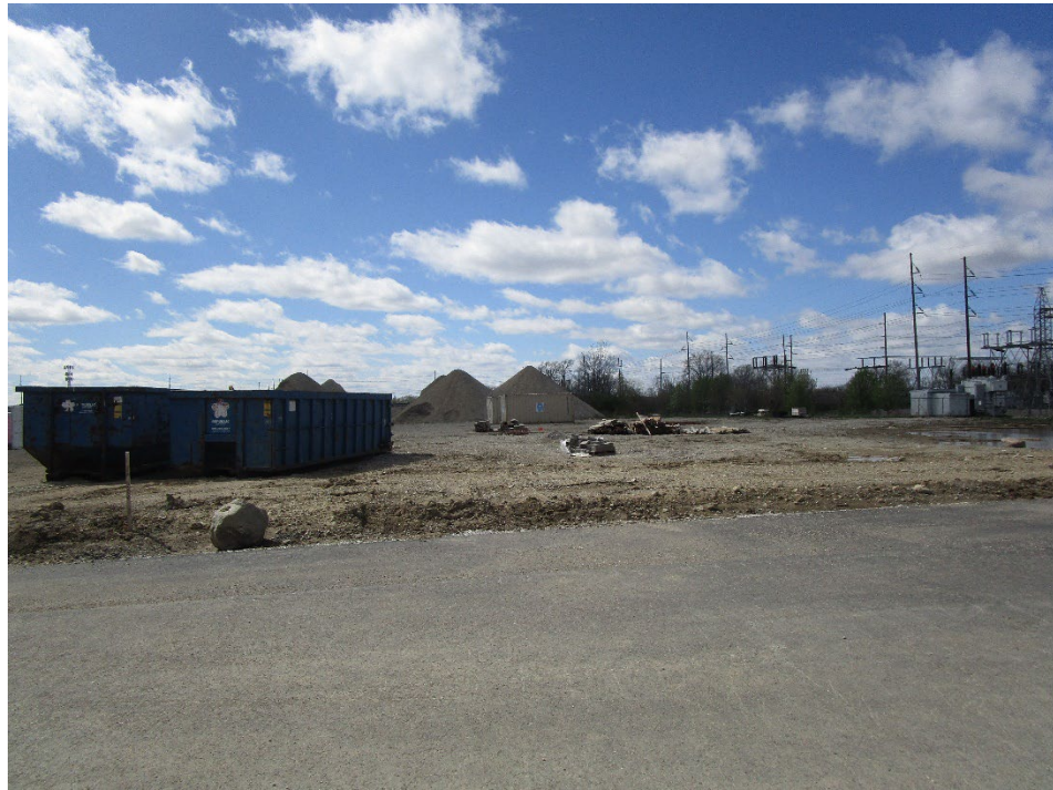
View of site looking northwest across Fintail Drive
