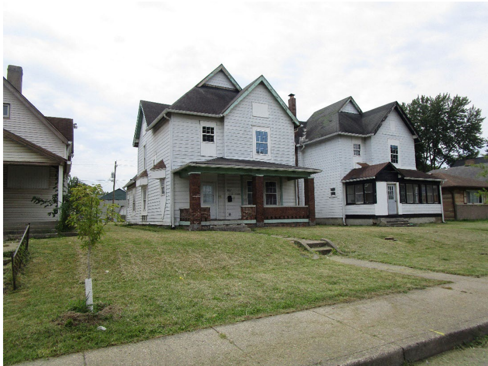
View of existing dwelling (1635 Woodlawn Avenue) looking south
