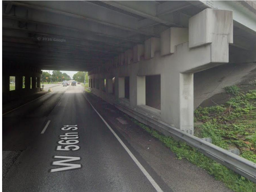
Photo 9: Southern Portion of 56 th Street Between Subject Site and Lafayette Road (July 2024)
