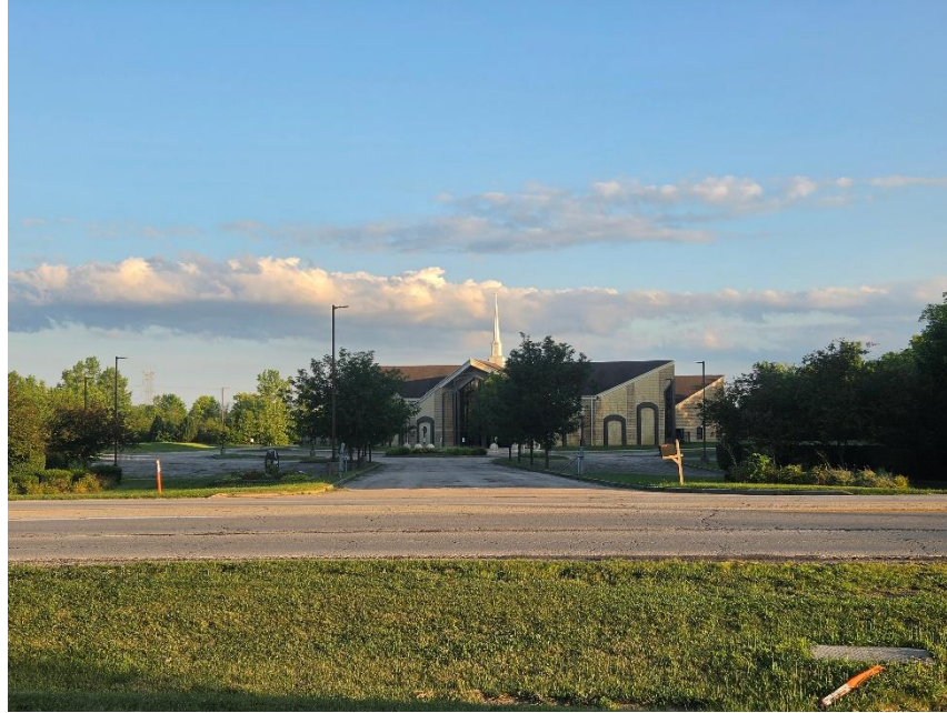
Photo 1: Subject Site Viewed from North
