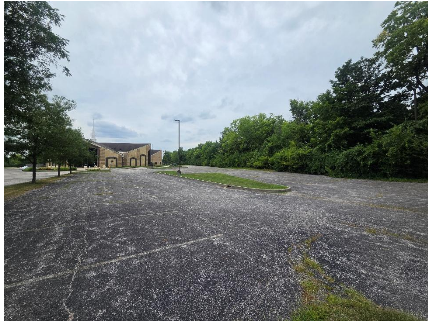
Photo 3: Existing Parking Area Viewed from North
