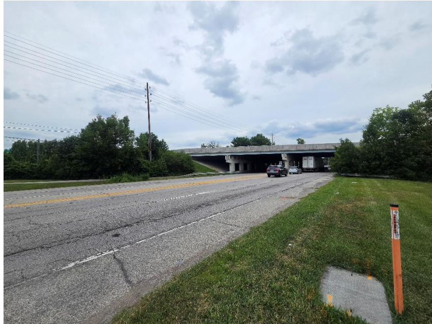
Photo 7: 56 th Frontage to East of Access Driveway
