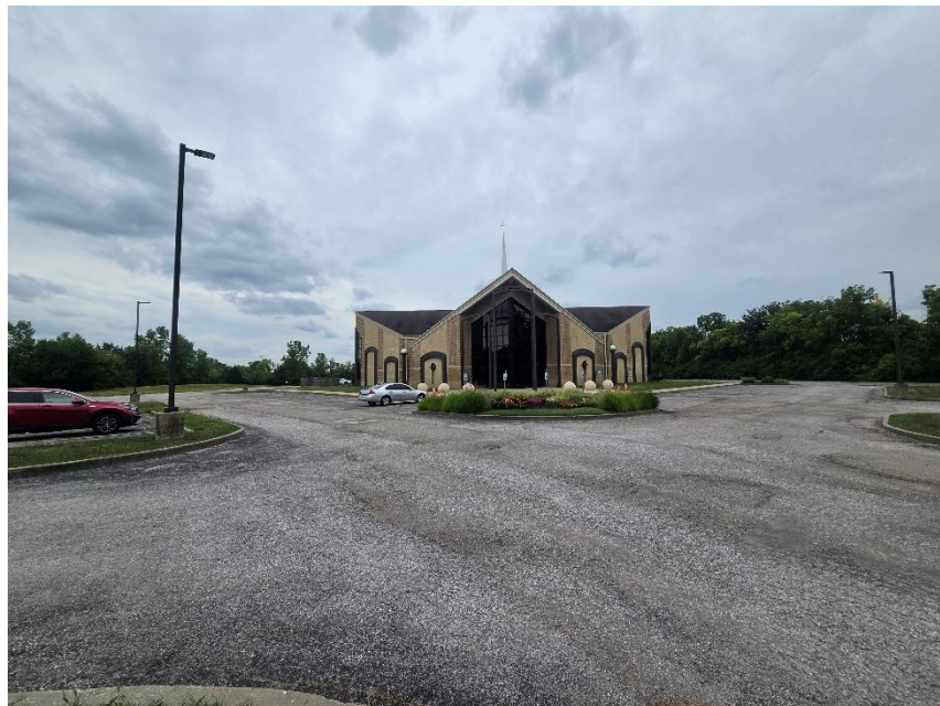
Photo 2: Existing Church Viewed from North
