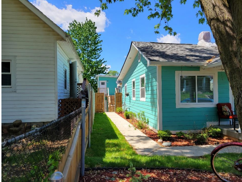
Photo 3: Southern Setback of Primary Residence + New Deck and Accessory Structure
