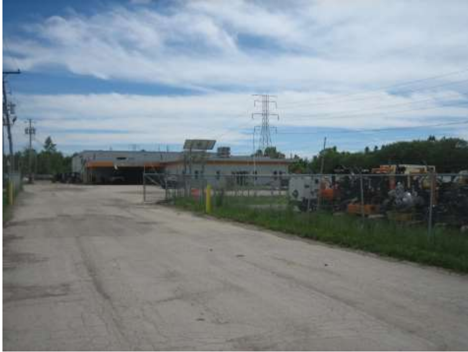
Subject site main entrance and building, looking south
