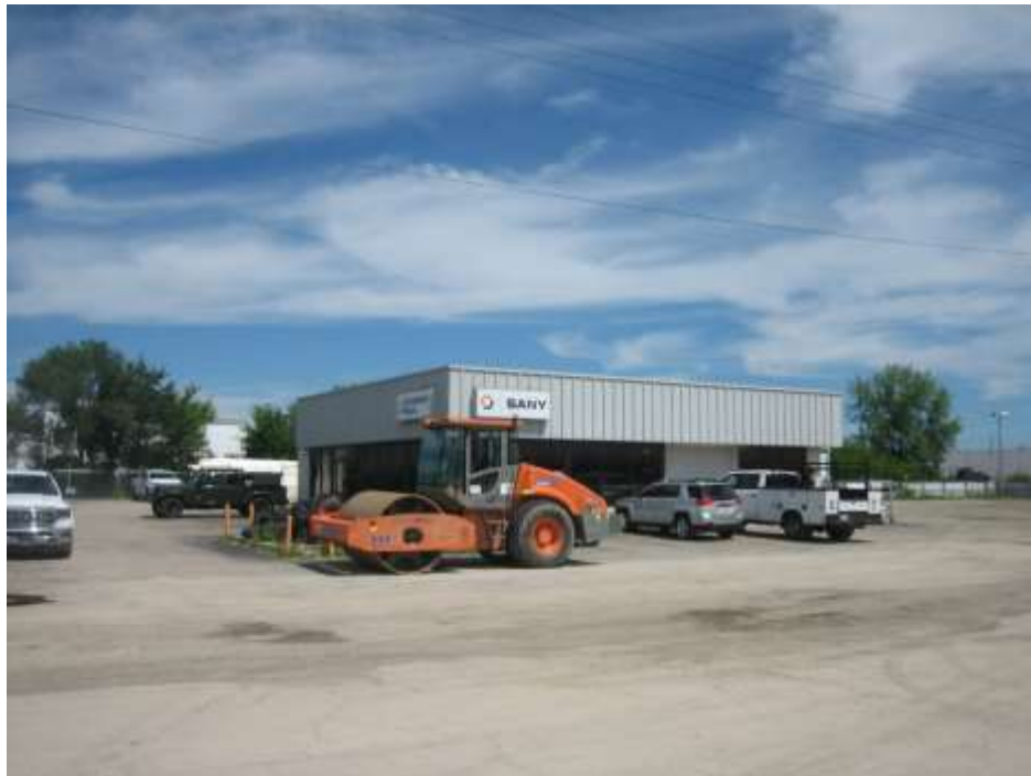
Subject site second parcel and building, looking southeast
