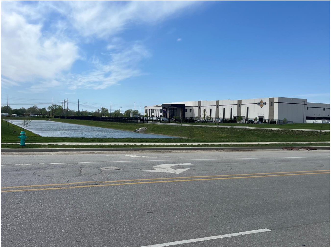
Photo 2: Adjacent property on western side of Fintail Drive
