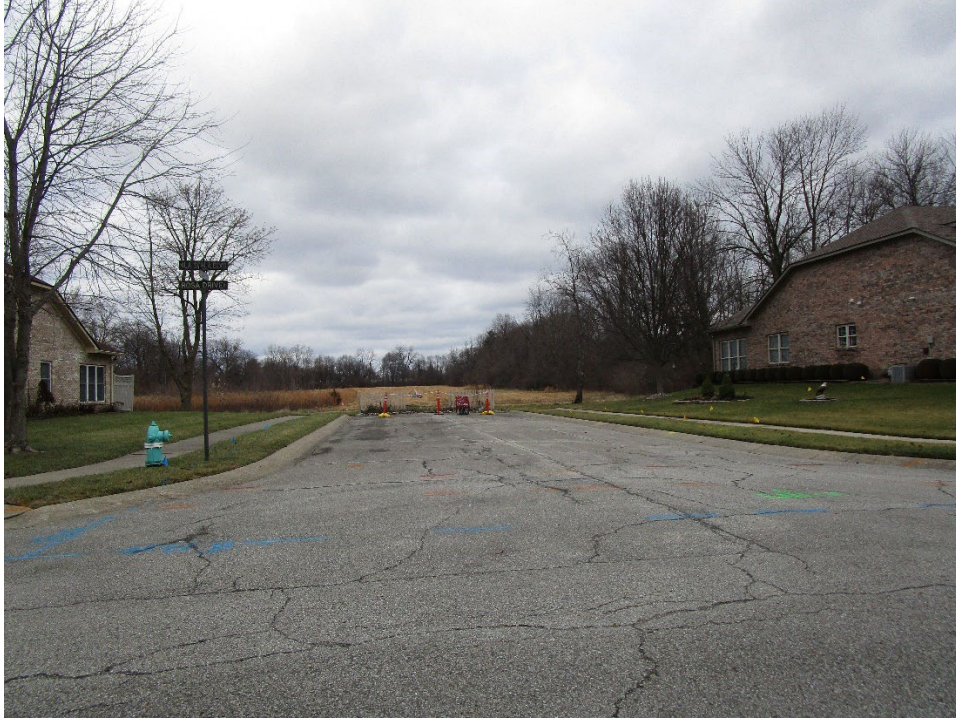
View of site looking north along Lasacala Boulevard
