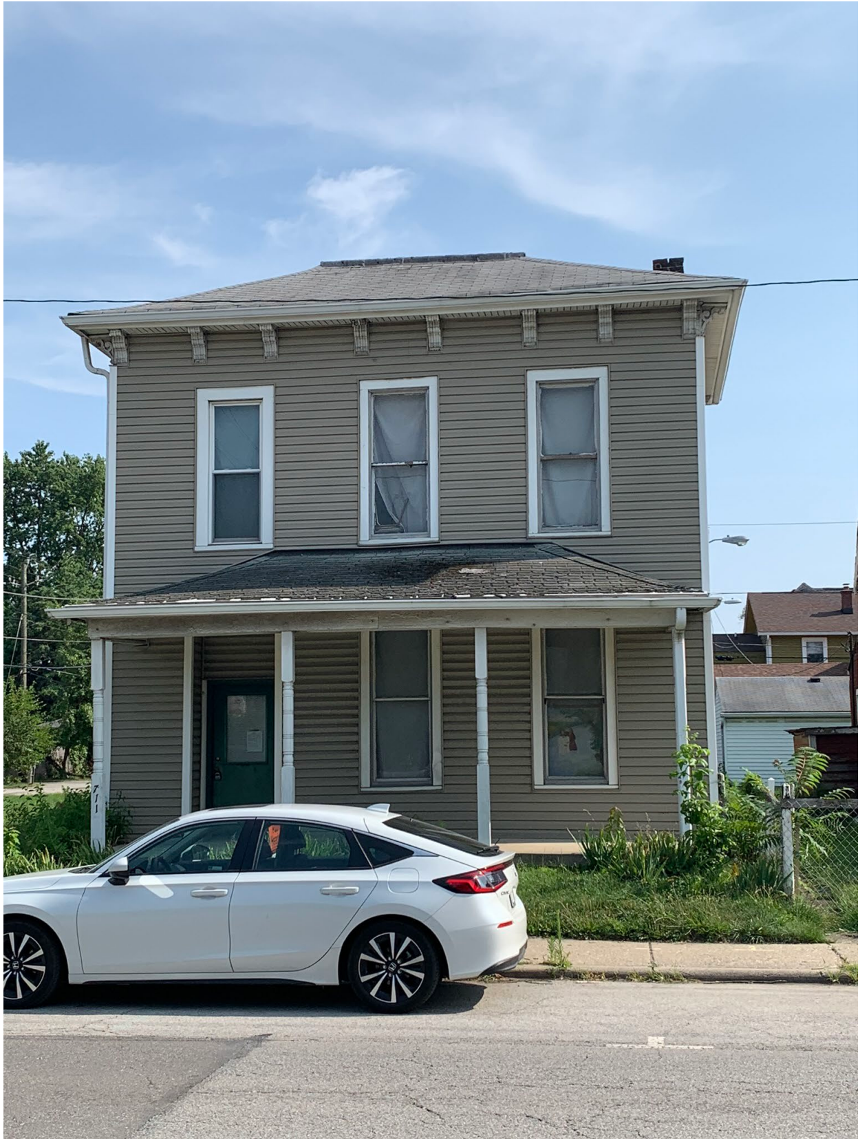
Existing structure at 707 East McCarty Street
