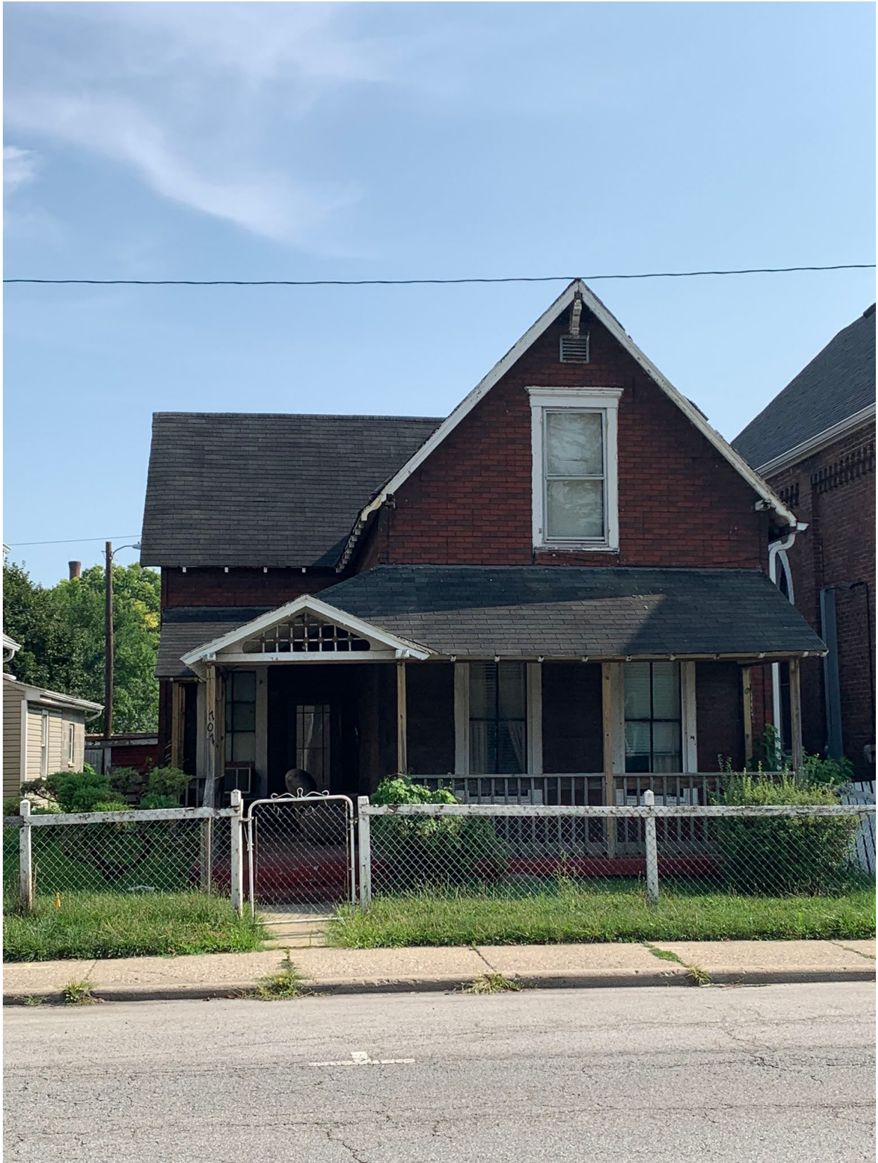
Existing structure at 707 East McCarty Street
