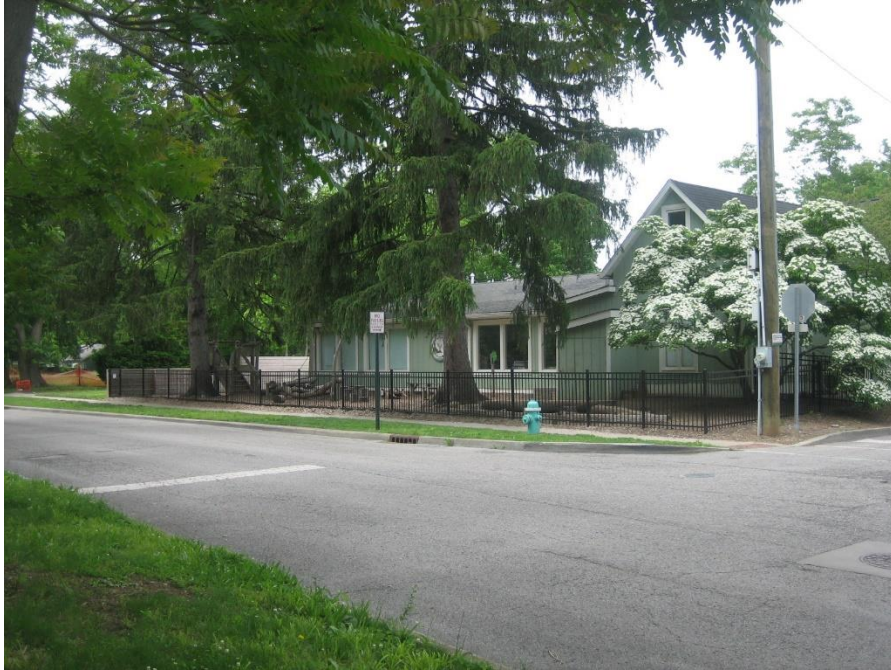
Subject site, looking southwest.
