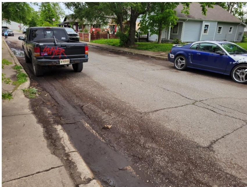
Photo 4: Adjacent Property to Southeast
