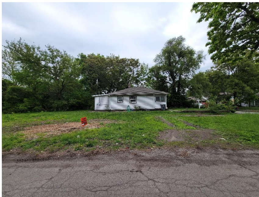
Photo 2: Subject Residence Viewed from West
