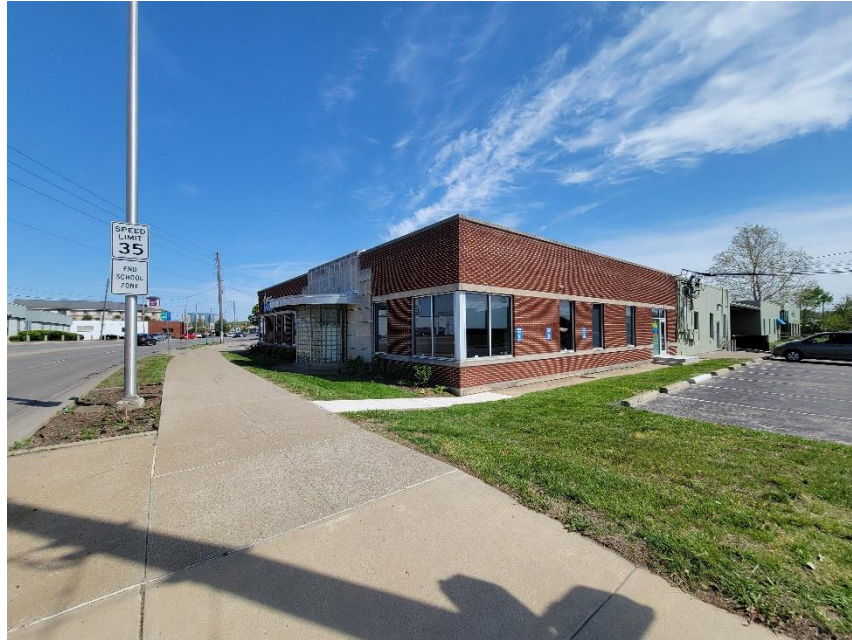
Photo 3: Subject Site Viewed from Northwest
