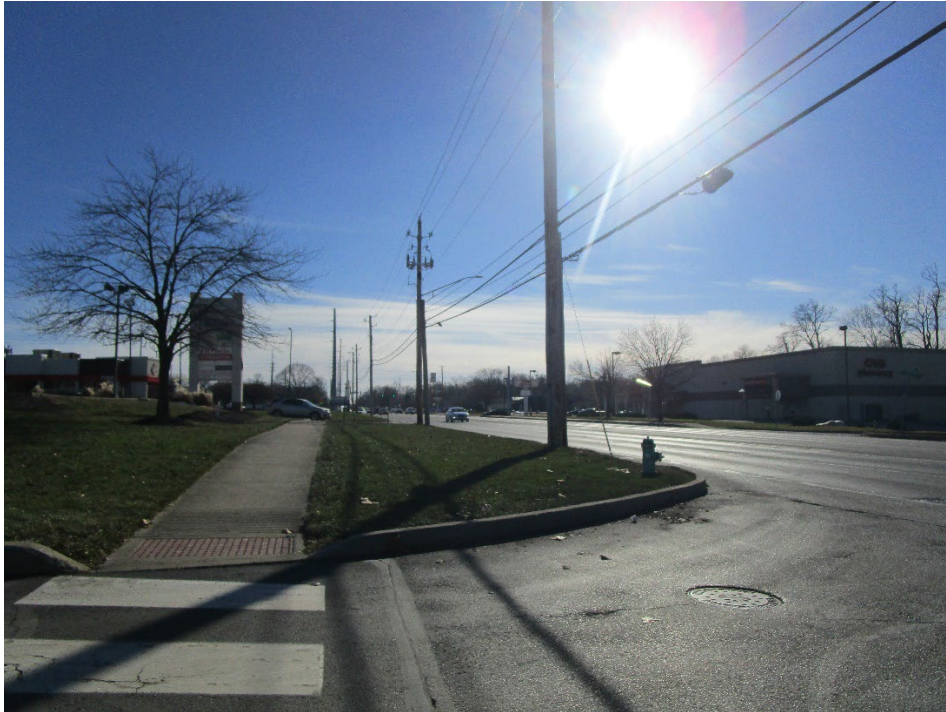
View looking south along Madison Avenue
