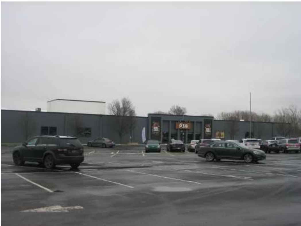
Existing subject site building, looking southeast.
